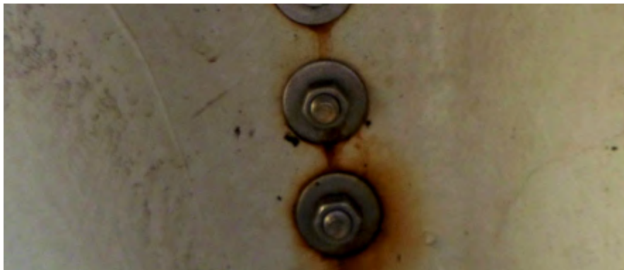
The chain plate bolts on a sailing yacht with some visual signs of corrosion. We can be pretty sure there's some crevice corrosion happening along the shank of the bolt. Deck fastenings should be re-bedded every 10 years to ensure the stainless steel is sealed from water ingress and potential corrosion.
