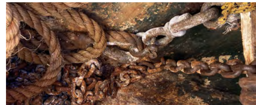
A very corroded anchor chain. It cannot reasonably be relied on to provide a secure anchoring. Failure of the anchoring system can result in vessel and third-party vessel damage, can result in injury. Basic owner routine inspections should have identified the problem and recorded it in the maintenance log as an urgent repair.
